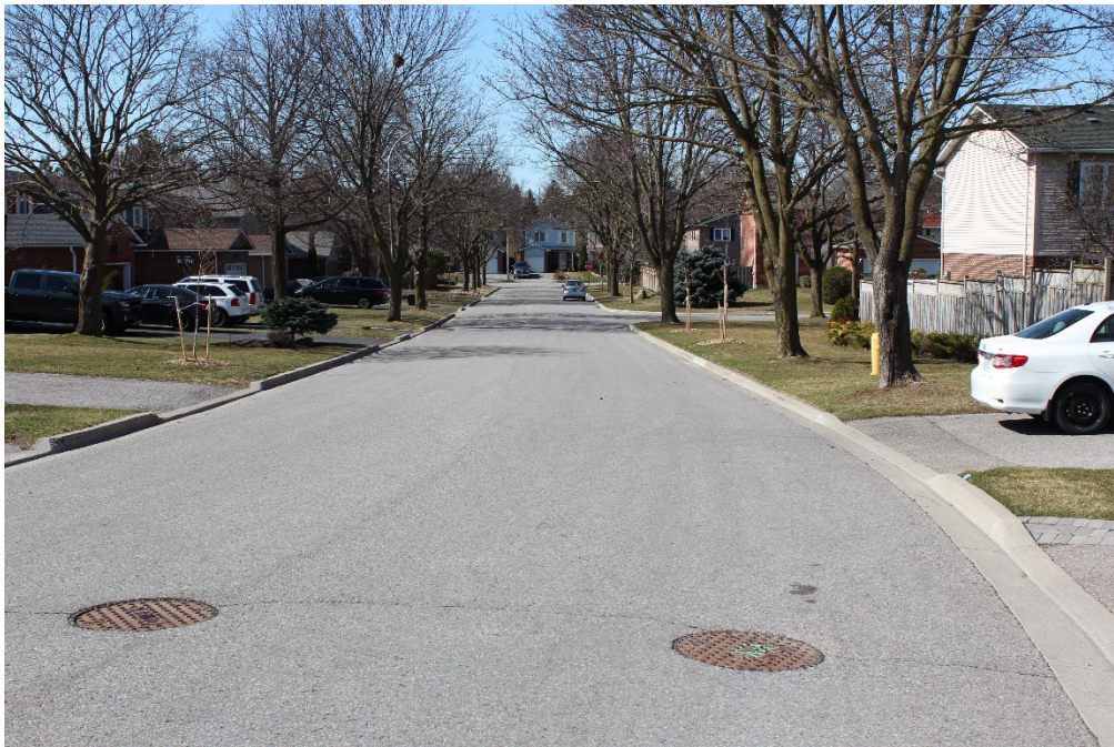
Figure 13 A photo of a road in Good condition
