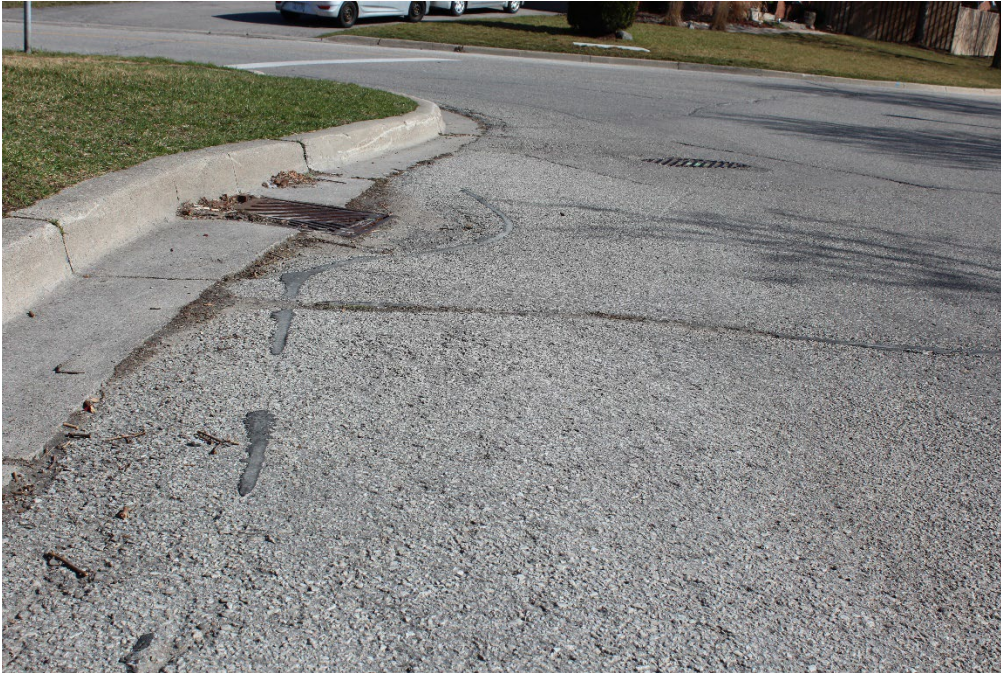
Figure 14 A photo of a road in Fair condition
