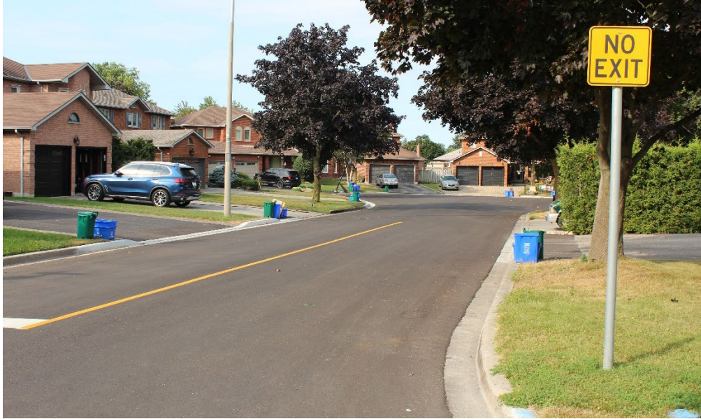
Figure 12 A photo of a road in Very Good condition
