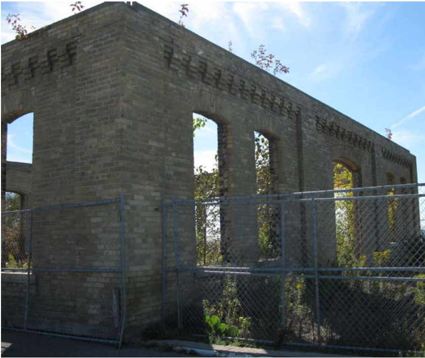
Pumphouse building view from the north west side
