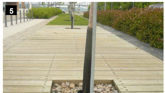
Surface materials would be enhanced to accentuate the prominence of the Waterfront Trail.
