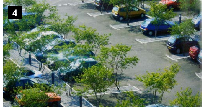
4 Existing surface parking lots would be enhanced to incorporate pedestrian walkways and tree plantings.
