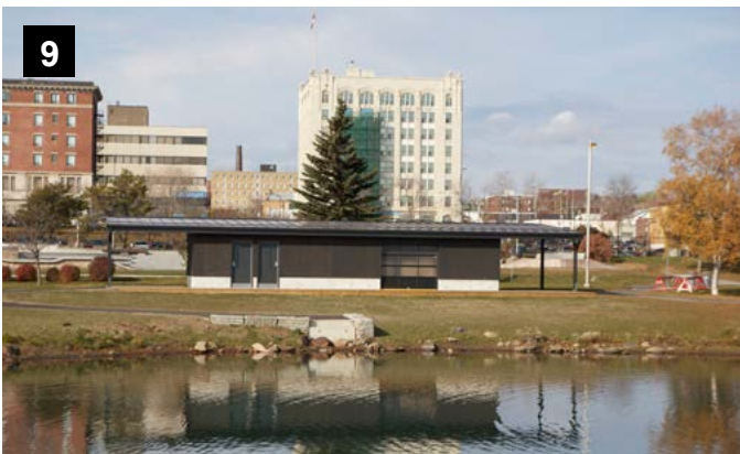
Year-round washrooms could be provided in locations where park or waterfront features are utilized throughout the winter months.
